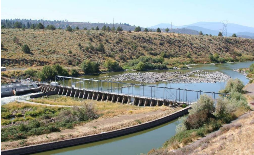
Figure 3-10. Photo of Link River Dam looking upstream. Spillway and fish ladder (fishway) are on the far left and the Eastside hydropower bay on the right side foreground. The reef is upstream of the dam. The two channels that were blasted through the reef are located on each side of the reef near the shoreline.
