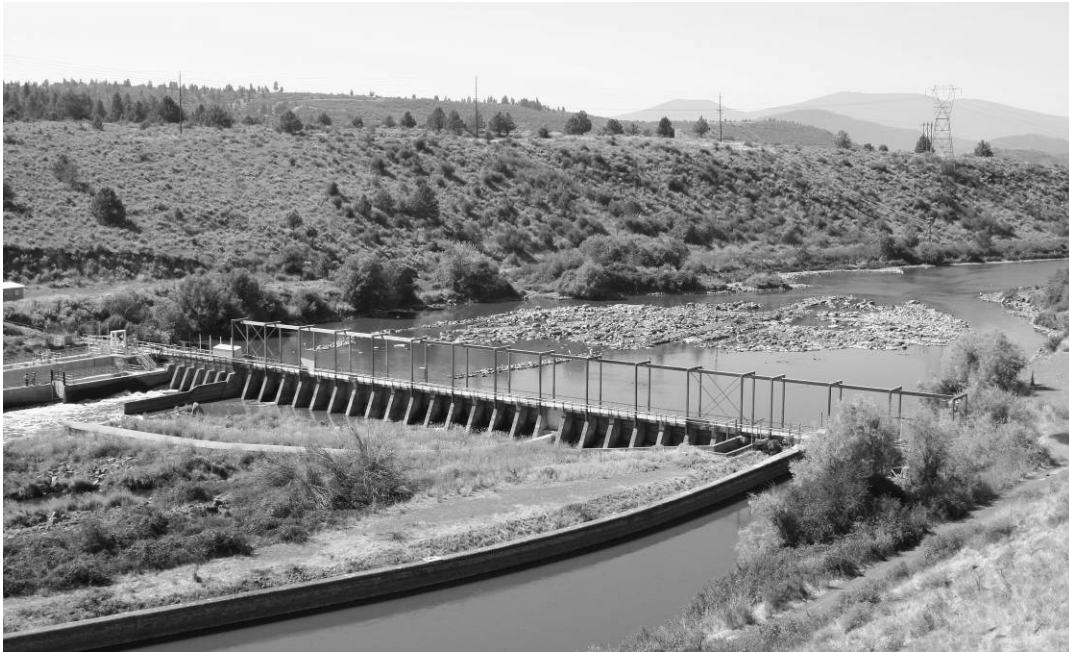
Figure 2. Photo of Link River Dam. Spill gates and fishway are on the far left and the Eastside hydropower bay on the right side. The reef is upstream of the dam. The two channels that were blasted through the reef are located on each side of the reef near the shoreline.
