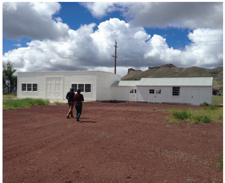
Under alternative C, the preferred alternative, the carpenter shop would be rehabilitated to serve as the unit's primary visitor contact facility. Photo: NPS.
